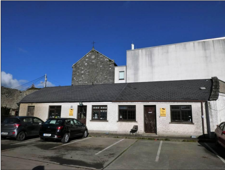
Plate 3 The northern outbuilding will be demolished during the construction of the proposed development. The proposal includes a market area complete with awnings for this section of the site.
